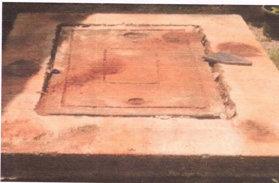
The Rainwater Harvesting System with ground water recharge has been installed
